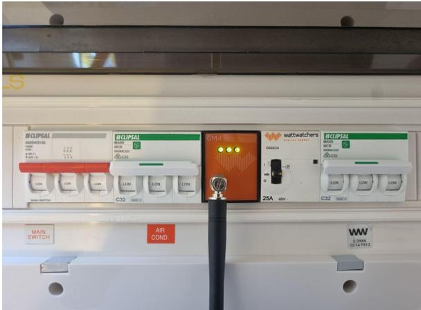
**NOTE:** The new 4G antenna is specifically designed for 3G/4G, but external high gain antennas (HGA) may be a better option for sites with low signal quality and only a few days of data can determine whether the HGA is working well or not. If 3 green lights do not appear with the HGA installed, remove it and try the 4G antenna provided then reboot the device.
